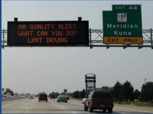
Dynamic Message Signs display messages to motorists, warning of hazards & providing information.
